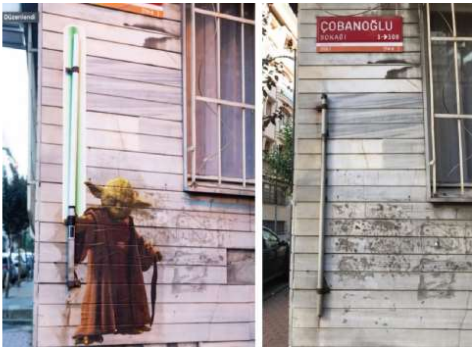
Figure 4.11 Rainspouts are repaired visibly by P13 and other association C members.
