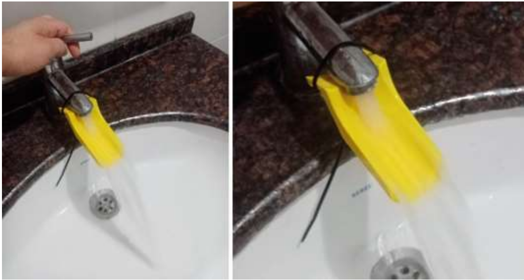
Figure 4.16 Yellow 3D printed plastic piece to fix the bathroom faucet by P15.
